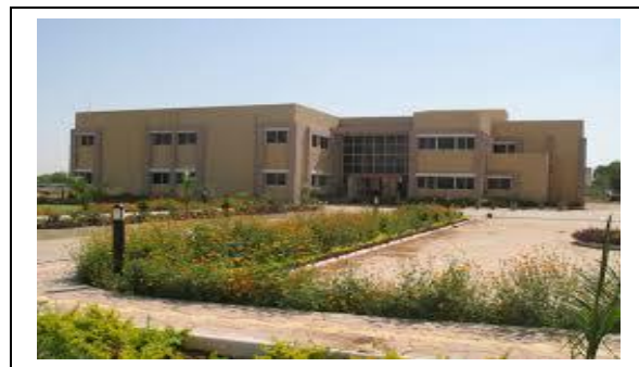
Renewable energy institute ,Dantiwada
